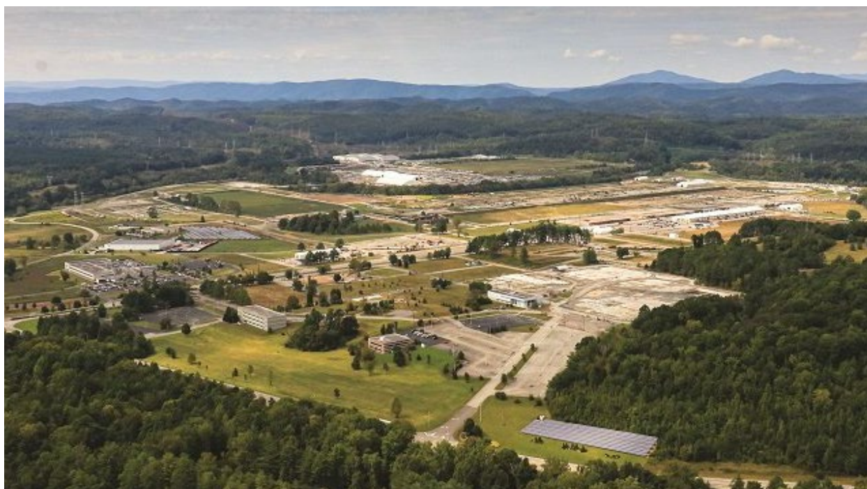
Figure 1.9. Aerial view of East Tennessee Technology Park
