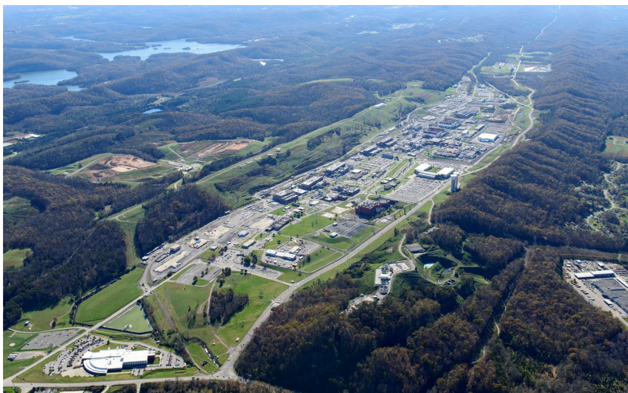
Figure 1.8. Aerial view of the Y-12 National Security Complex
